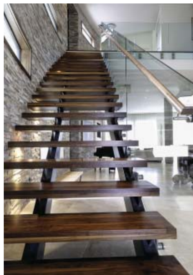
As one walks through the front door, you are immediately drawn to the unique staircase. A set of commercial heavy duty standoffs hold the 2" thick glass that lines the staircase. Glass was used so as to not obstruct the visibility of the 24' high stacked brick wall. The thick wood planks used on the stairs are of a beautiful Caribbean Koa supported by a painted metal structure.
