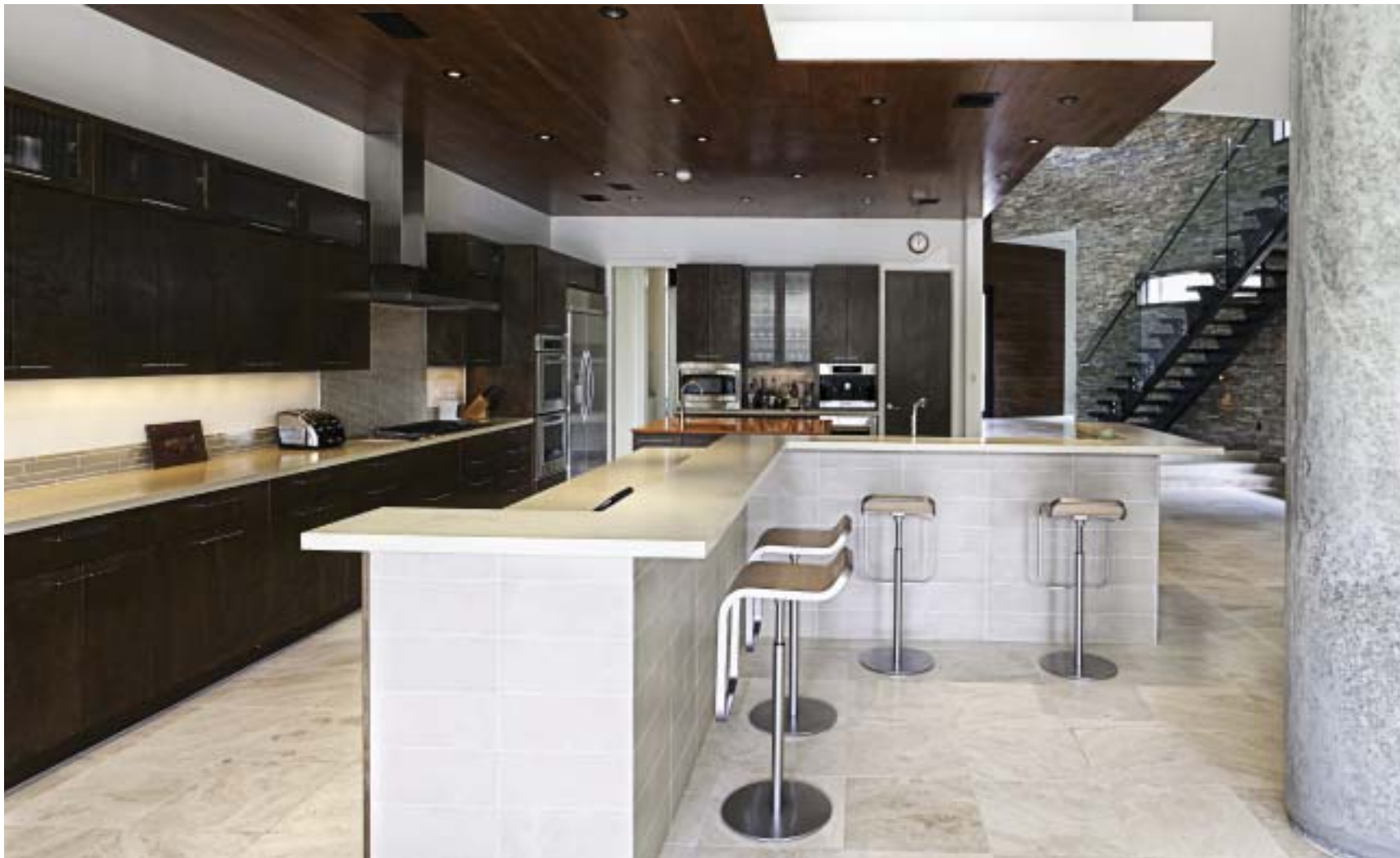
Since the house had such an open floor plan, I wanted the kitchen to stand out and make a statement. Therefore, the ceiling was dropped and mahogany wood was installed to give it coziness and warmth. The beige kitchen counters are Quartz and the bright orange island was added for color. A linear porcelain tile was used on the vertical surface for durability purposes, since the counter is a very popular space for guests to hang out. Travertine flooring was used throughout the first floor making the space warm, natural and giving it great movement. The principal structural support is a massive 18" concrete column that stands in the middle of the open floor plan, which adds a certain raw beauty to the otherwise polished space. Bar-height chairs are from Design Within Reach.
